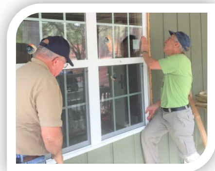
John and Jay installing
