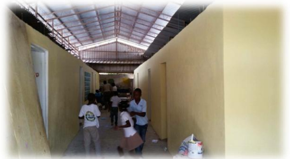
PICTURE OF THE NEW SCHOOL WALLS!
